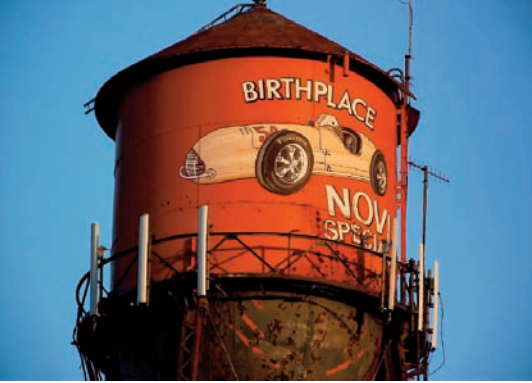
Novi Special Water Tower
