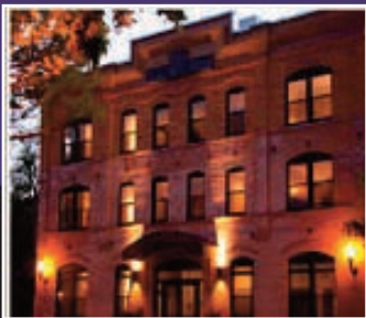
Chauvet Converted Hotel Glen Ellyn, California
